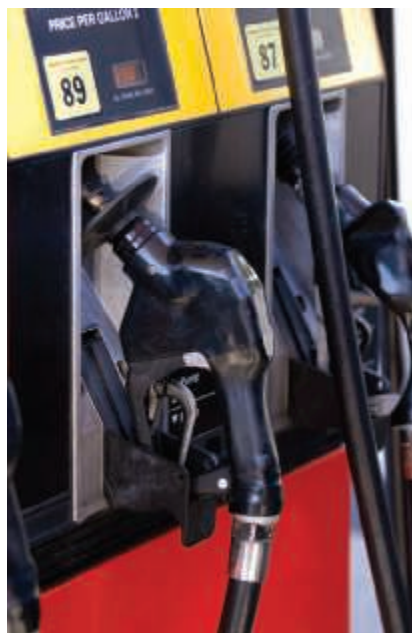
▲ Figure 24.6 Octane rating. The octane rating of gasoline measures its resistance to knocking when burned in an engine. The octane rating of the gasoline in the foreground is 89.
